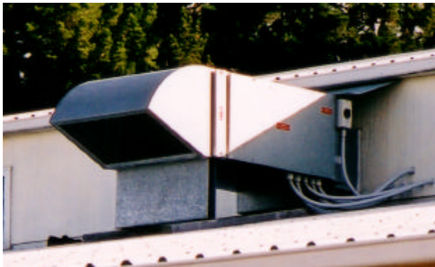
Weatherproof supply air handler
